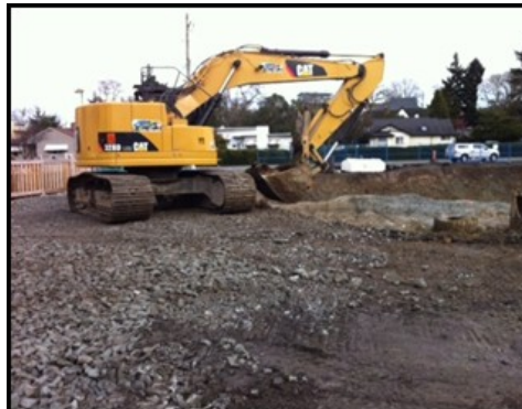
Construction begins at 35 Gorge Road
